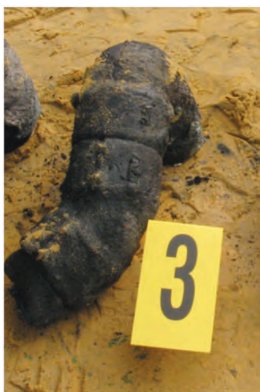
Figure 51 Fill pipe elbow of tank 3 — elbow is significantly fire affected, as shown in Figure 48
