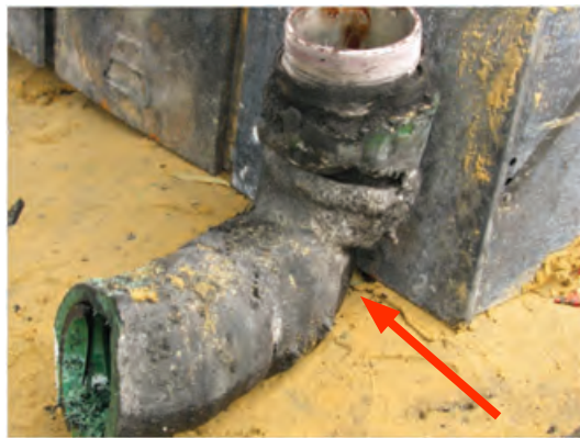
Figure 54 Fill pipe elbow of tank 4 — elbow section is significantly fire affected, as shown in Figure 64
