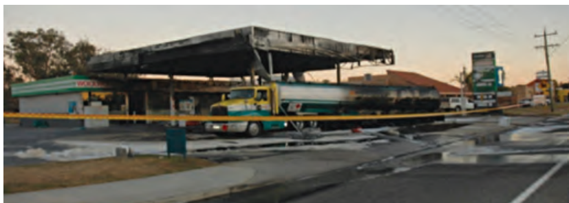
Figure 17 Position of the fuel tanker in relation to the service station canopy [photograph courtesy of FESA]
