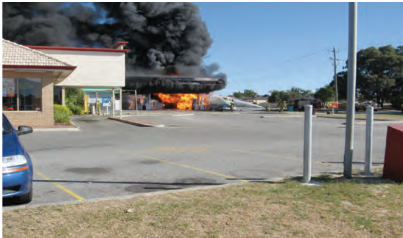
Figure 15 Spread of fire from the tanker to service station canopy and building [photograph courtesy of Department of Environment and Conservation]
