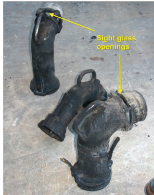
Figure 33 Underground tank fill elbows. Central unit is the vapour recovery elbow
