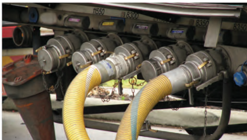
Figure 59 Typical tanker outlet valves in the open position (i.e. lever on right hand side of valve, parallel to hose)
