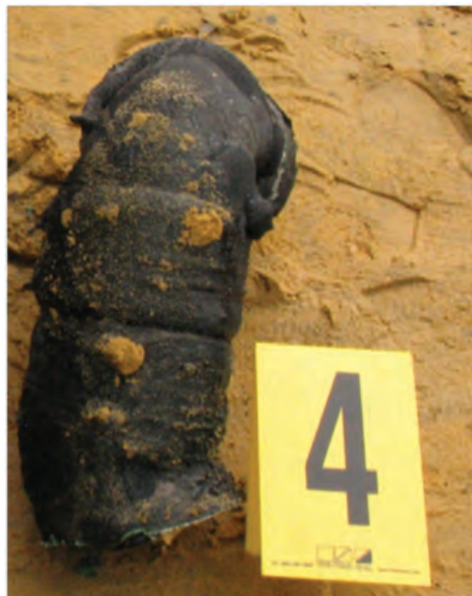
Figure 55 Fill pipe elbow of tank 4 — elbow section is significantly fire affected
