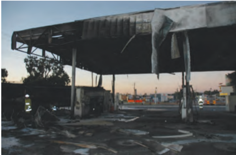
Figure 22 Extensive damage to the service station canopy and fuel dispensers
