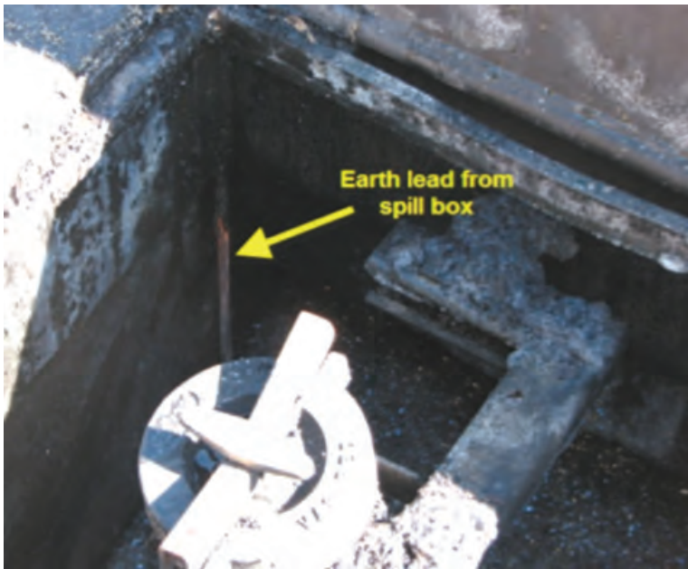
Figure 23 Vapour recovery connection point
