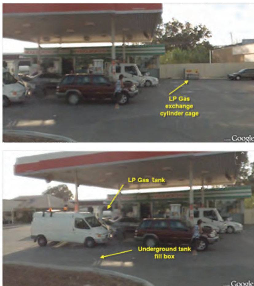
Figure 3 Street views of the Woolworths Petrol Maddington service station [images from Google Earth]
