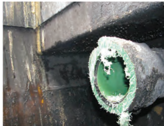
Figure 44 Tank 1 fill pipe inside containment sump — fill pipe is in good condition
