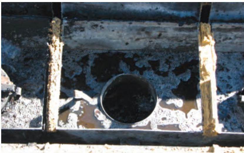
Figure 25 Tank 3 fill point with missing fill point
